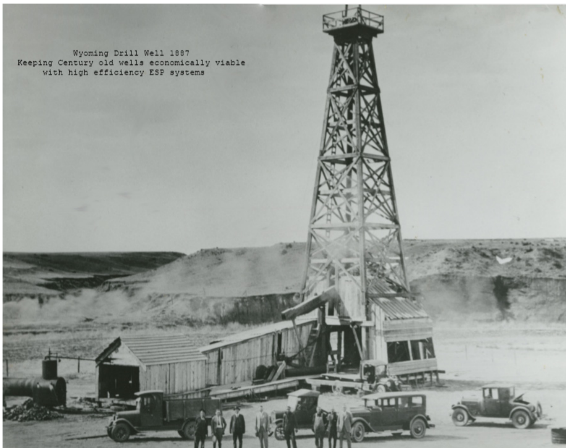
PowerSave high-efficiency ESPs are being used to extend the economic life of wells in Wyoming drilled as early as 1887.
