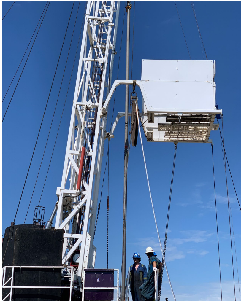
Replacing the pumpjack and rod-lift equipment with a PowerSave high-efficiency ESP with a PMM not only saved money, it also increased oil production by 70%.
